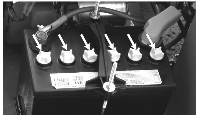
Figure 7.7 - Battery Fluid Level
