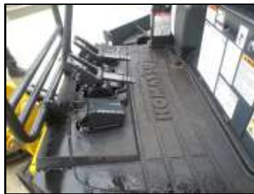
Operators cabin flooring.
