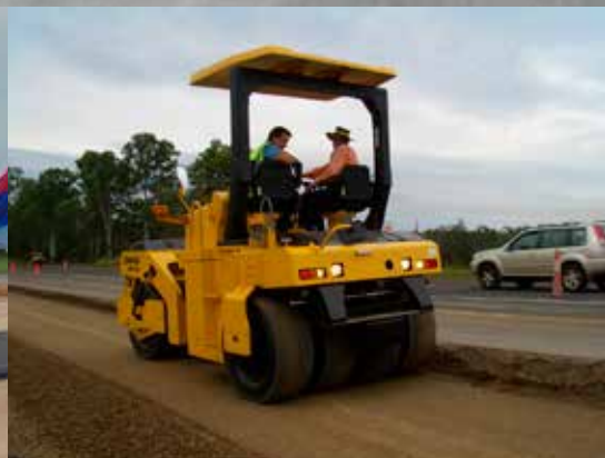
Soil subbase, Australia
