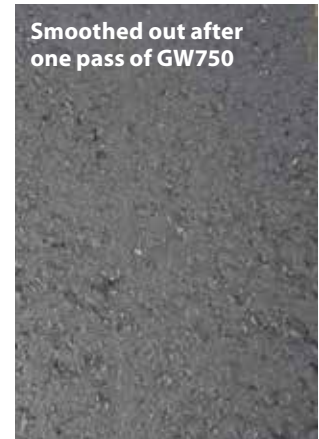
Fig 4. Remove hairline cracks from HMA pavement
