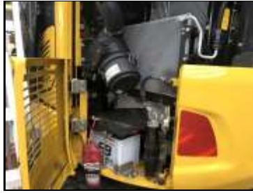
Battery, radiator header tank and oil cooler.
