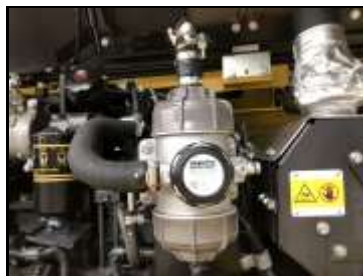
Crankcase ventilation filter and surrounding components
