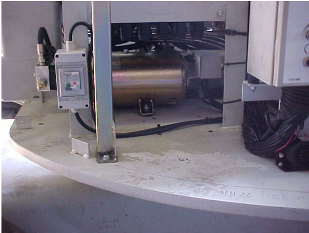
Photo 11 - Built-in generator and
