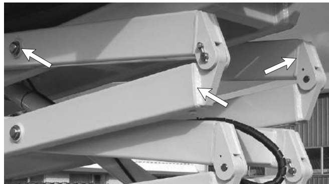
Figure 7.19 - Structural Damage and Welds
