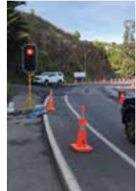
Operator can now stand safely away from the eSTOP. Use handset to change signals as required
