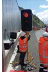
Once facing oncoming traffic, tighten locking screw
