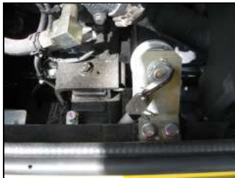
Battery isolation switch.
