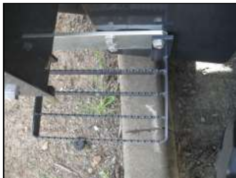
Clearance to back edge of rung on rear maintenance step RHS.
