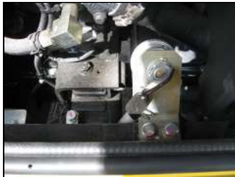
Battery isolation switch
