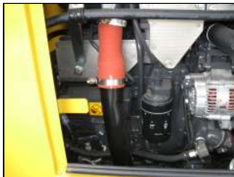
Compressed air hose(turbo to aftercooler).
