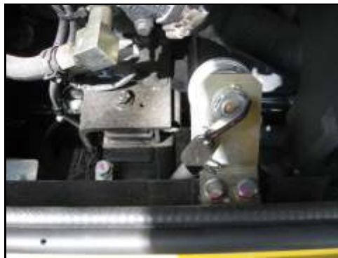
Battery isolation switch.
