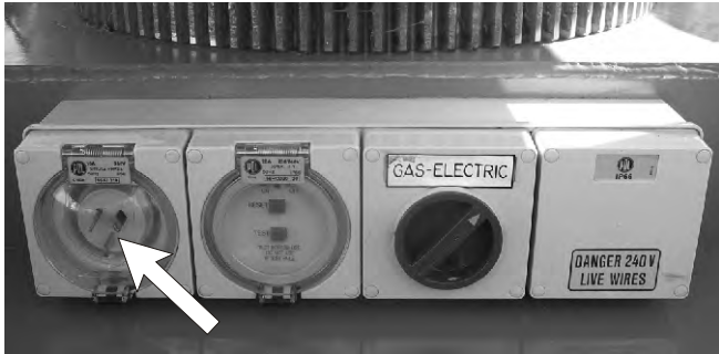
Figure 11.11 - AC Power Input Connector
