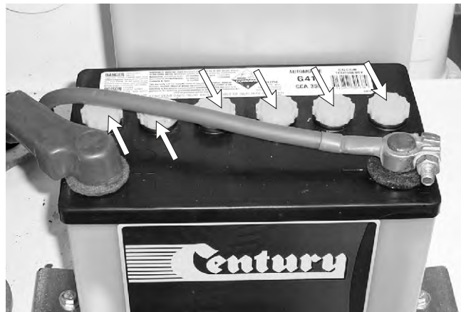
Figure 7.7 - Battery Fluid Level
