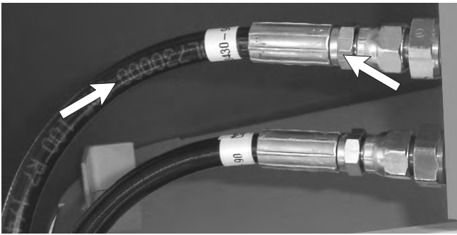
Figure 7.10 - Hydraulic Oil Leaks At Fittings And Hoses
