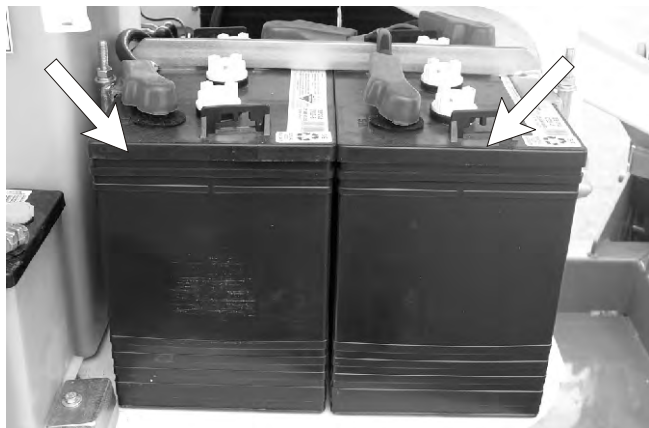
Figure 11.6 - Two DC Motor Batteries (Petrol/Diesel Engine Side)
