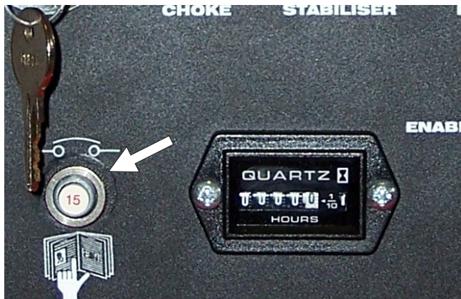
Figure 5.2 - Main Circuit Breaker
