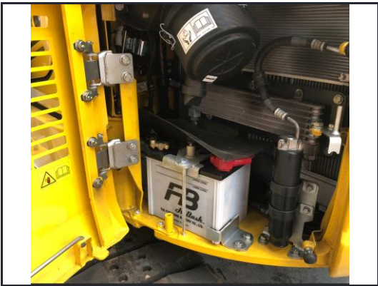
LHS service bay/battery box access
