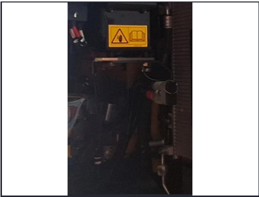
Warning decals installed.
