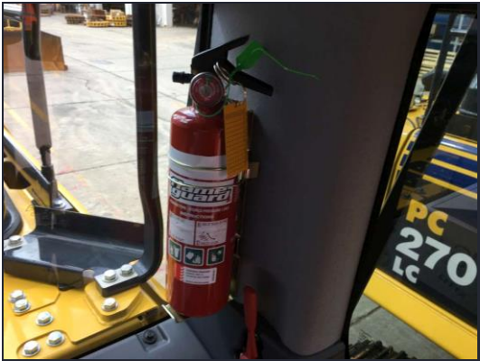
Portable fire extinguisher inside cabin.
