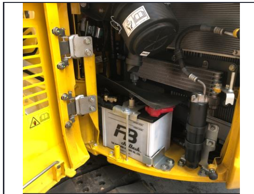
Battery box access
